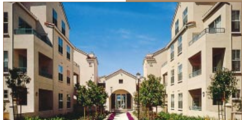
Avalon on the Alameda San Jose, CA
