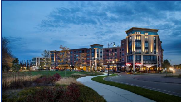
AVALON AT ASSEMBLY ROW SOMERVILLE, MA
